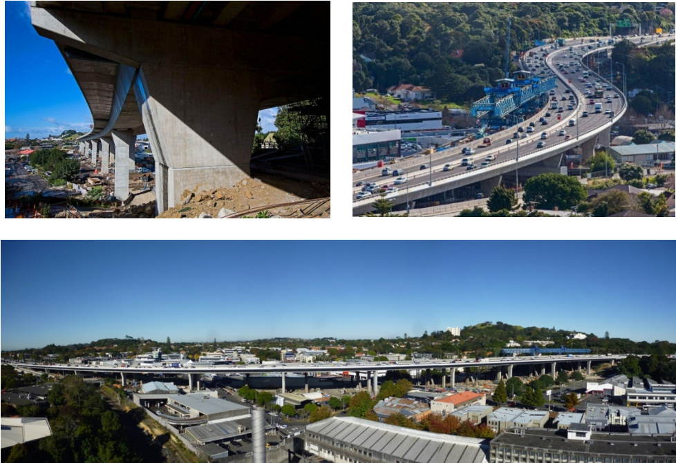
Figure 1. Views of Newmarket Viaduct [13].
