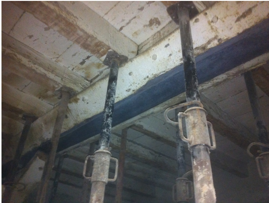
Figure 1: Applications of FRP strengthened timber beams.
