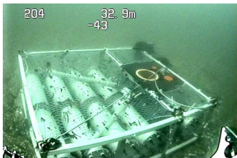
Fig. 2. FLOWBEC subsea frame deployed on the seabed in 33 m of water at the EMEC tidal energy test site. The image is taken from an ROV during recovery of the frame—the recovery bridles can be seen now laying across the frame prior to being lifted. This image was taken during the first deployment, (2012), before a rigid platform was added for the ROV to land on, to aid hooking the recovery bridle.
