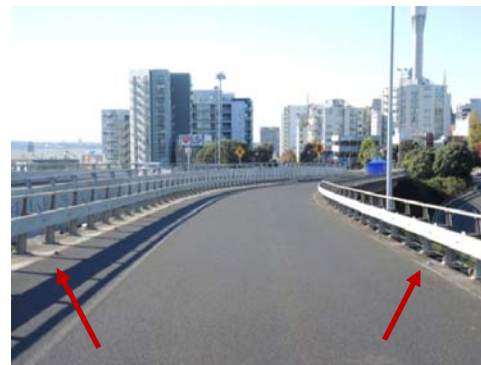
Figure 4. Accelerometers arranged along the bridge curbs.
