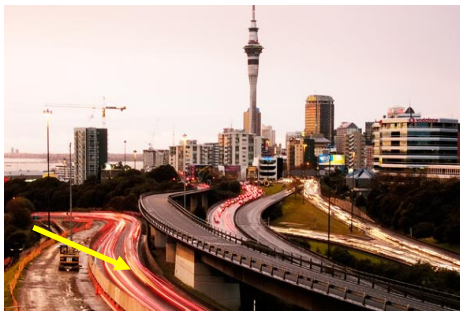
Figure 1. Aerial view of the Nelson St off-ramp bridge.
